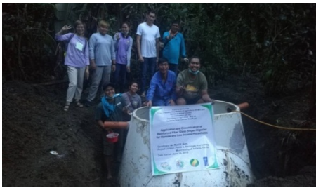
Completion of installing a digester
